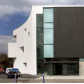
Front elevation Photo: Morley Von Sternberg
